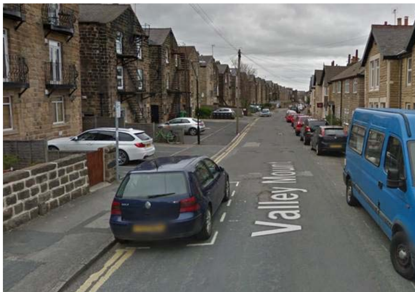
Photo showing existing disc parking space
